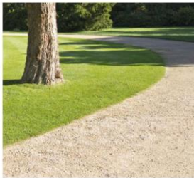
Example of compacted hoggin surface
